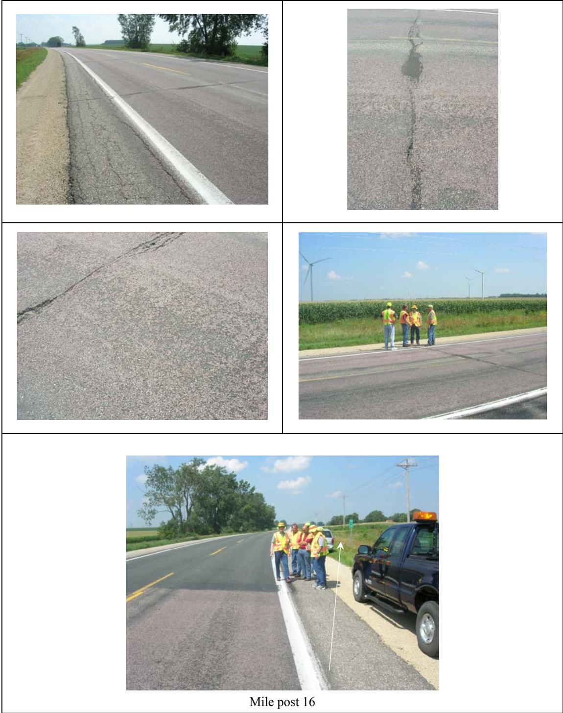
**Figure C.5. TH 56 sections with surface treatment applied in 2000 (built in 1995),
