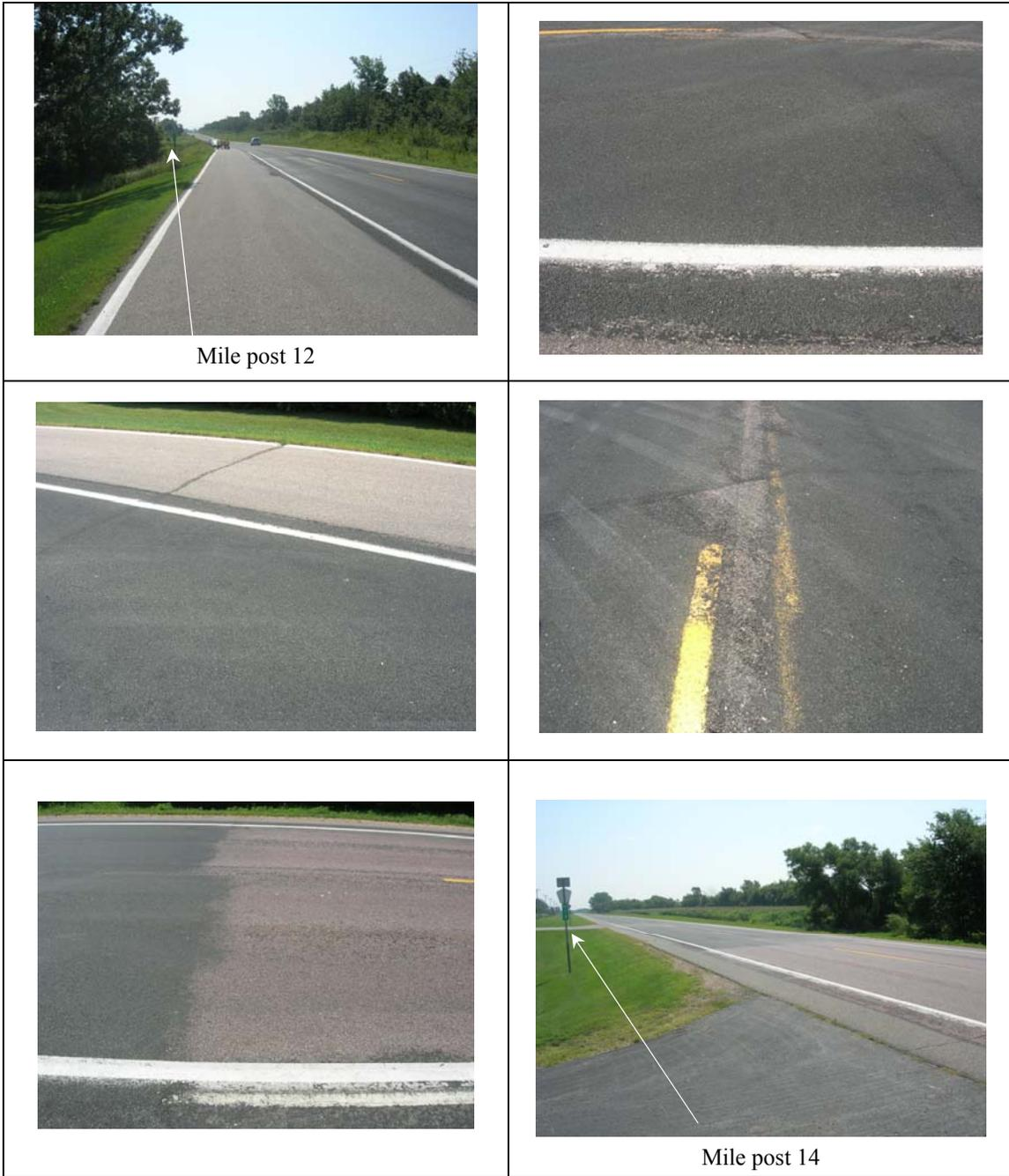
**Figure C.3. TH 56 sections with surface treatment applied in 2002 and 2001 (built in 1999), mile 12 to 13 and 13 to 14, respectively.**
