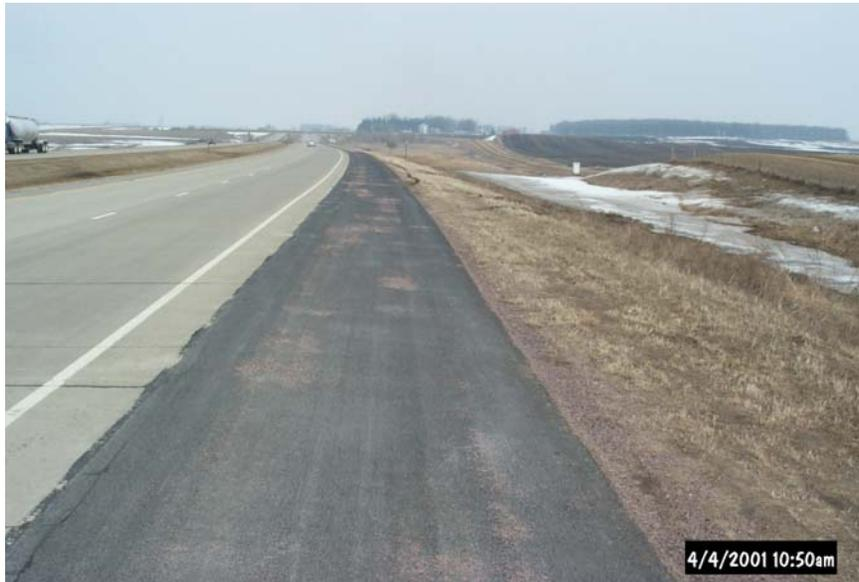
**Figure B.4. Shoulder seal coat I-35, R.P. 15-16**
